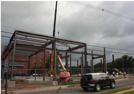
Steel Framing - Storrs Center
