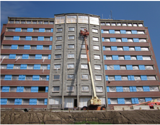
International Hall - midway through repairs July 7, 2011
