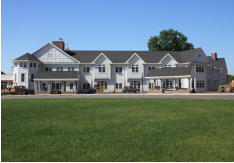
Primary School at the Fay School
