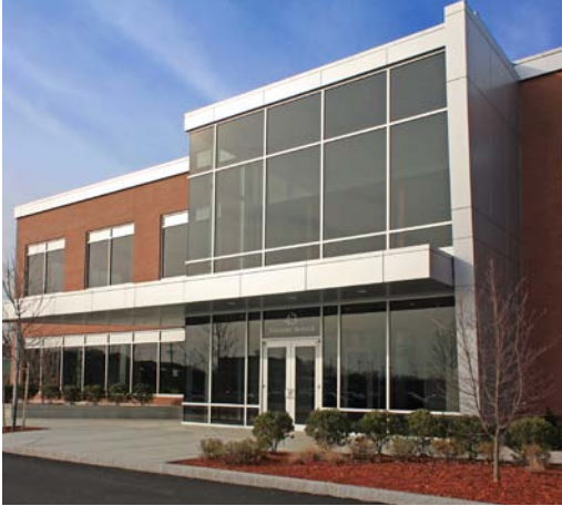
43 Foundry Avenue, CenterPoint Waltham, Massachusetts
