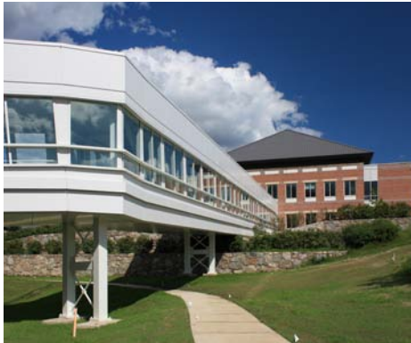
Bridge Connecting 65 and 75 Network Drive
