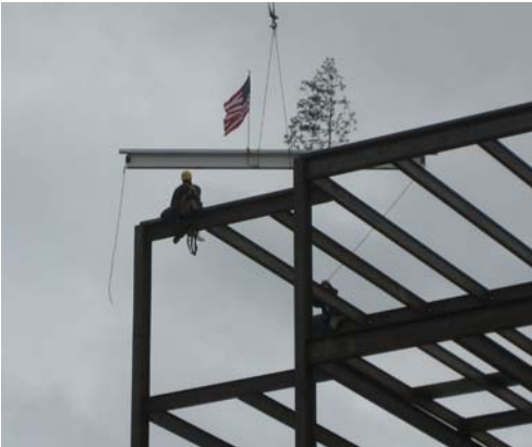
The beam is secured into place by steel workers.
